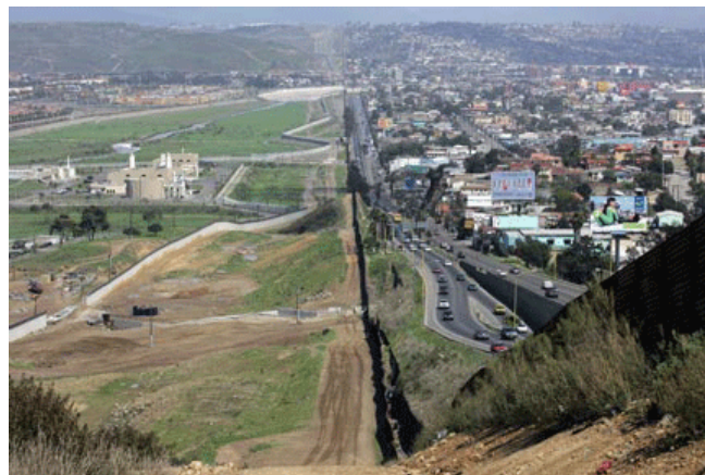
The DHS created a task group to provide cross-border communications interoperability by connecting communications centers in the United States and Mexico. Photo by Gerald L. Nino
